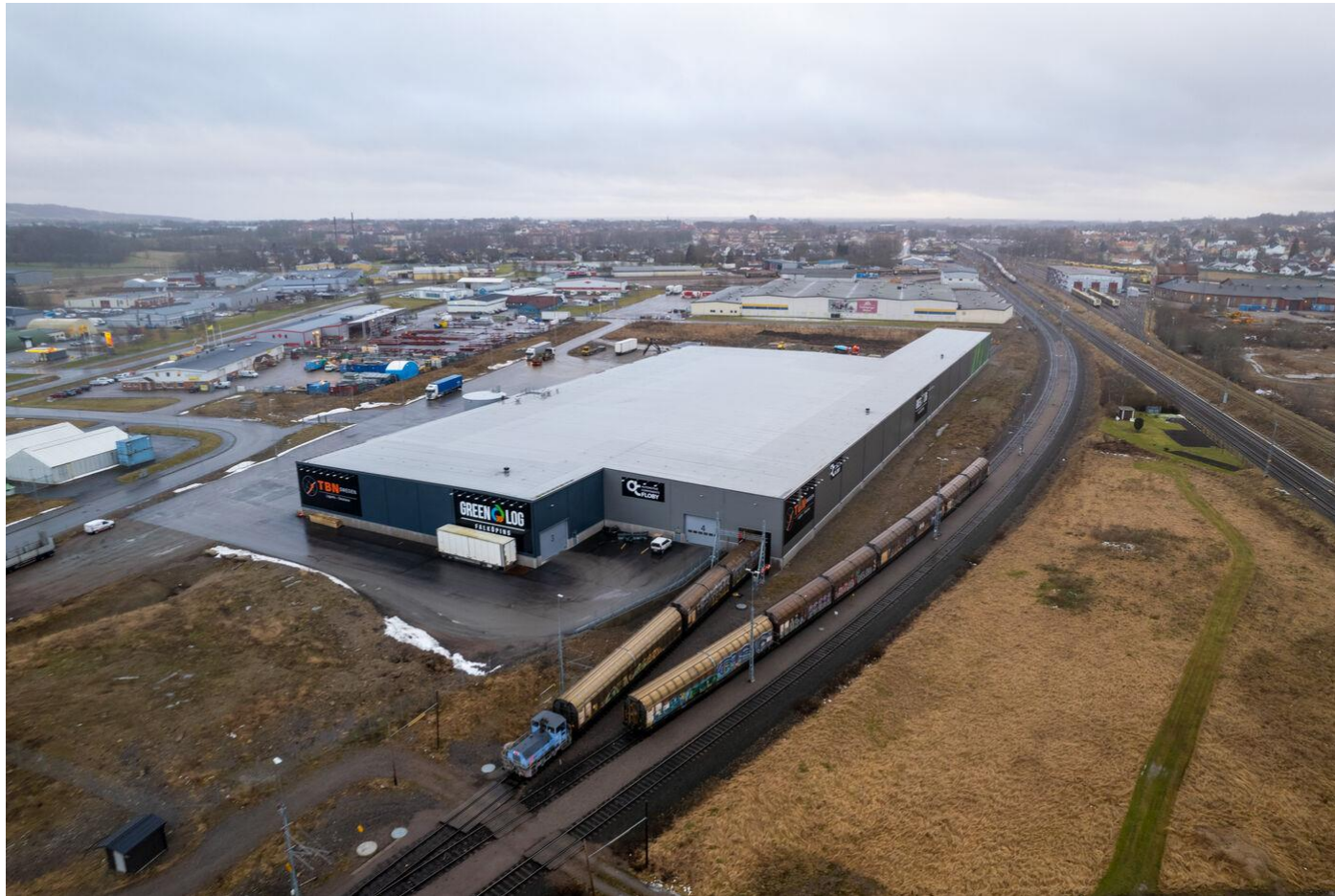
Multimodal terminal operations: rail-to-road transshipment in Sweden
